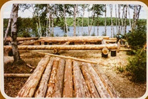
Above: In the foreground are the old telephone poles Doug floated as the foundation on which to rest logs. This photo also shows the small footprint of the 18x22-foot cabin.
