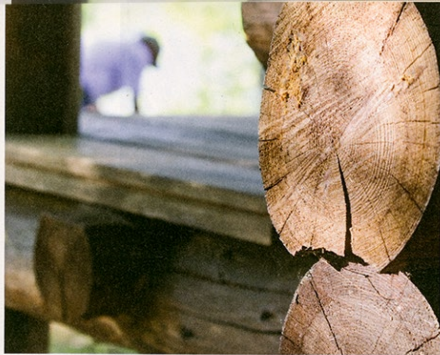
Above: In the foreground are the old telephone poles Doug floated as the foundation on which to rest logs. This photo also shows the small footprint of the 18x22-foot cabin.
