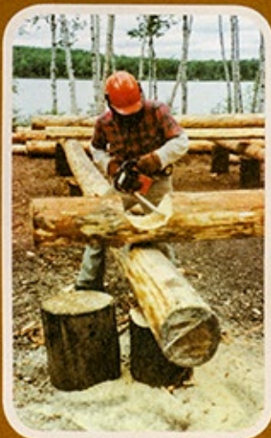
Above: In the foreground are the old telephone poles Doug floated as the foundation on which to rest logs. This photo also shows the small footprint of the 18x22-foot cabin.
